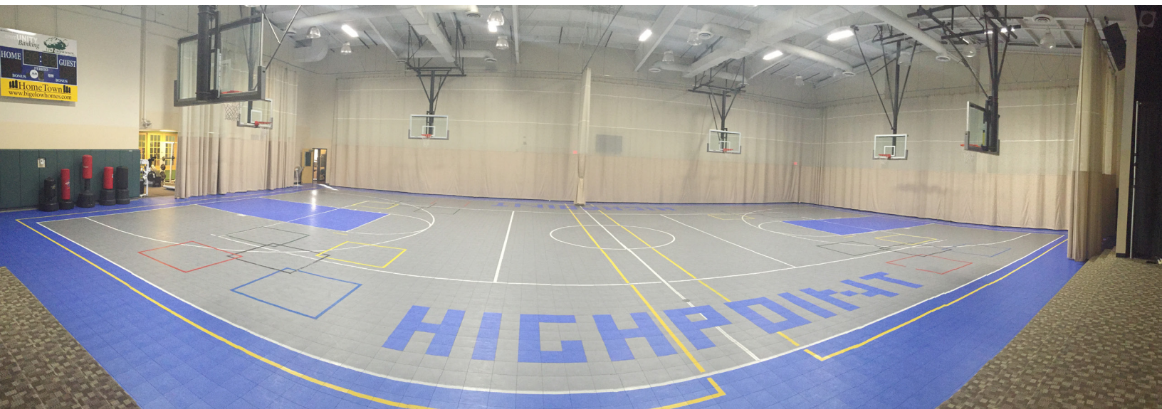
20 metal halide fixtures (460W each), replaced with 12 LightSource LS18 LED fixtures (150W each)
