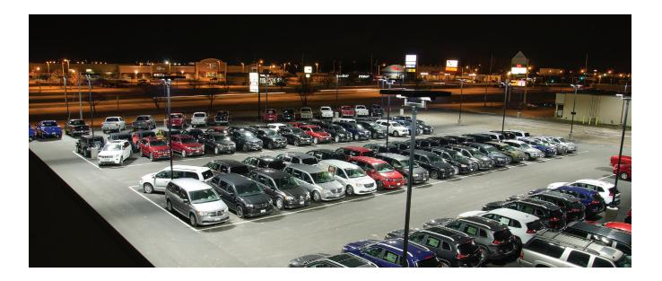
model T 600W fixtures are Dark-Sky compliant and provide exceptional light cut-off, which means less spill over onto adjacent property.
