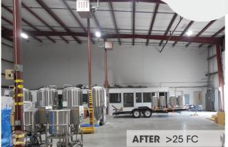
Smart operations. A **65% reduction in energy** was achieved in this loading bay by upgrading existing HID fixtures to energy efficient energybank LED OmegaLight™.
