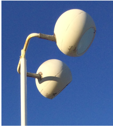
EXISTING Two - 1090W HID
